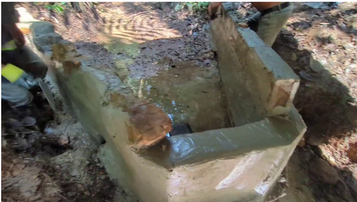
Figure 3.1. Concrete Block, Rock, and Cement Weir for the Eco-Libre Life-Line at Fruit Haven in Morona-Santiago, Ecuador (attribution: Boris Plotkin )
