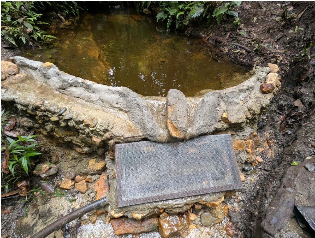
Figure 3.2. Rock and Cement Weir for the Eco-Libre Life-Line at Fruit Haven in Morona-Santiago, Ecuador (attribution: Vegan Beasts )
