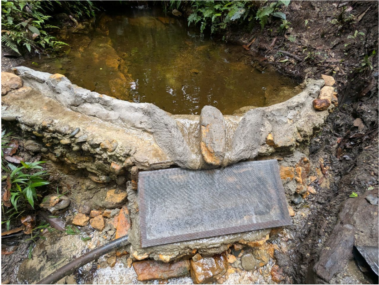
Figura 3.2. Rock and Cement Weir for the Eco-Libre Life-Line at Fruit Haven in Morona-Santiago, Ecuador (attribution: Vegan Beasts )
