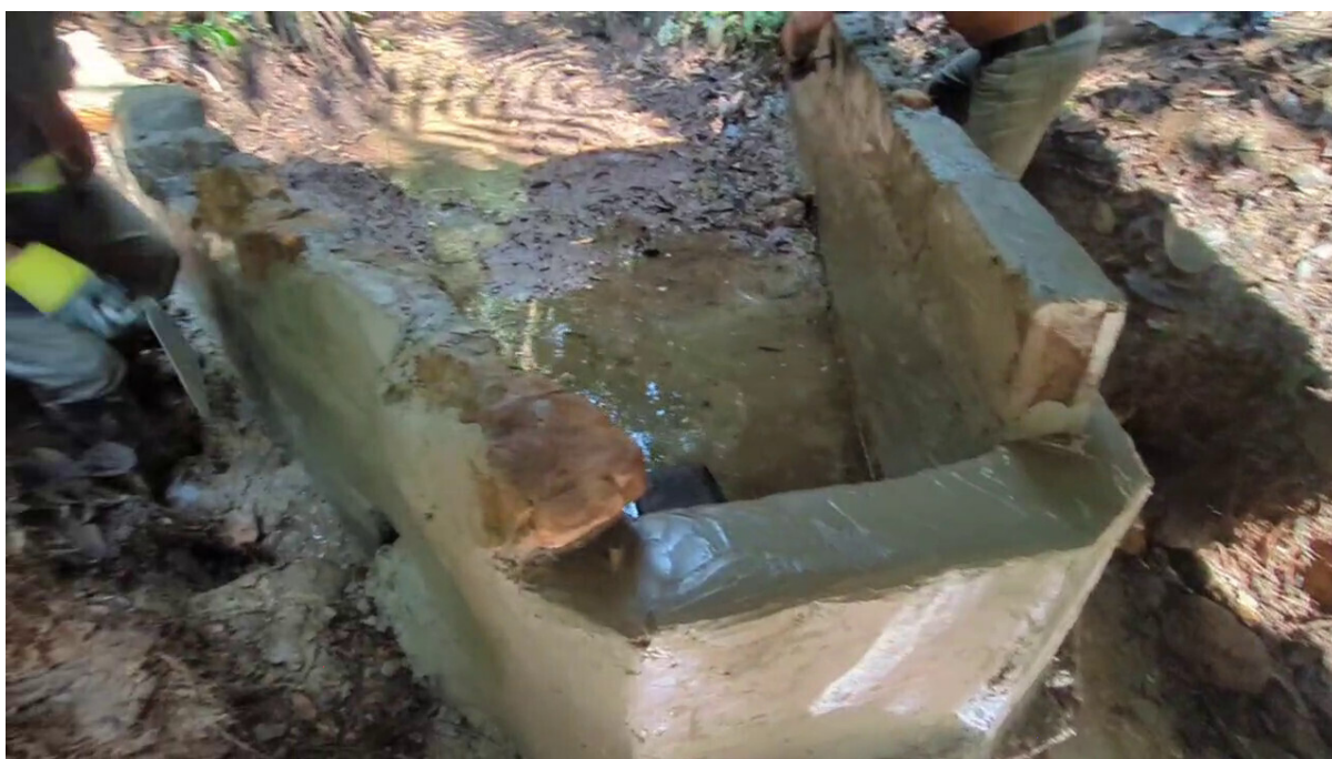
Figura 3.1. Concrete Block, Rock, and Cement Weir for the Eco-Libre Life-Line at Fruit Haven in Morona-Santiago, Ecuador (attribution: Boris Plotkin )
